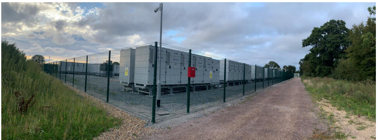
Plate 15.47: Example of a BESS Site
