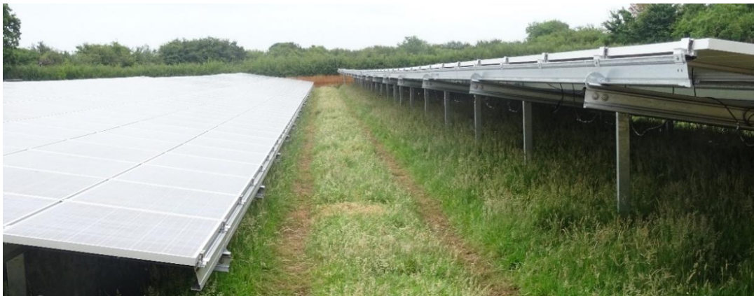
Plate 15.32: Part Installed Panels (Bentham Farm, Purton)
