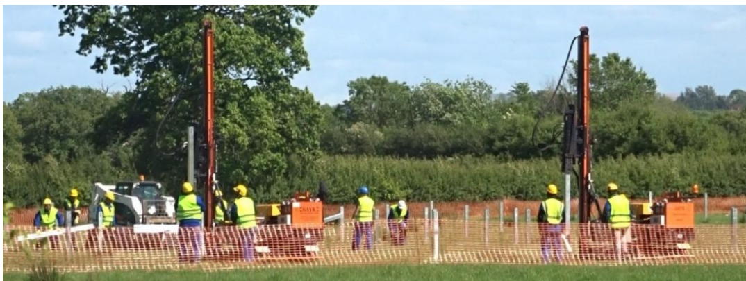
Plate 15.30: Mounting Structure Piles being Installed
