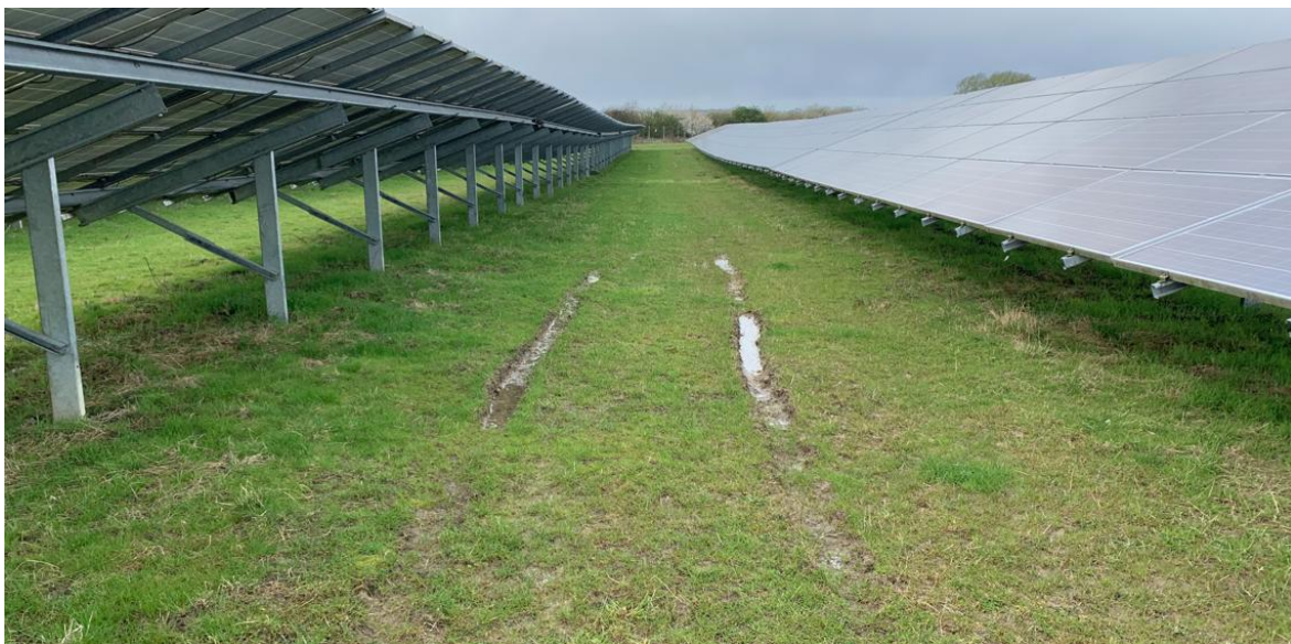
Plate 15.52: Example of Minor Ruts Caused by Vehicles
