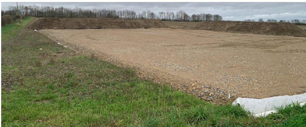
Plate 15.22: Example Construction Compound (being built)
