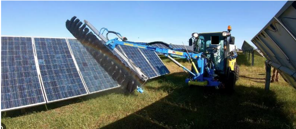
Plate 15.51: Cleaning of Solar Modules
